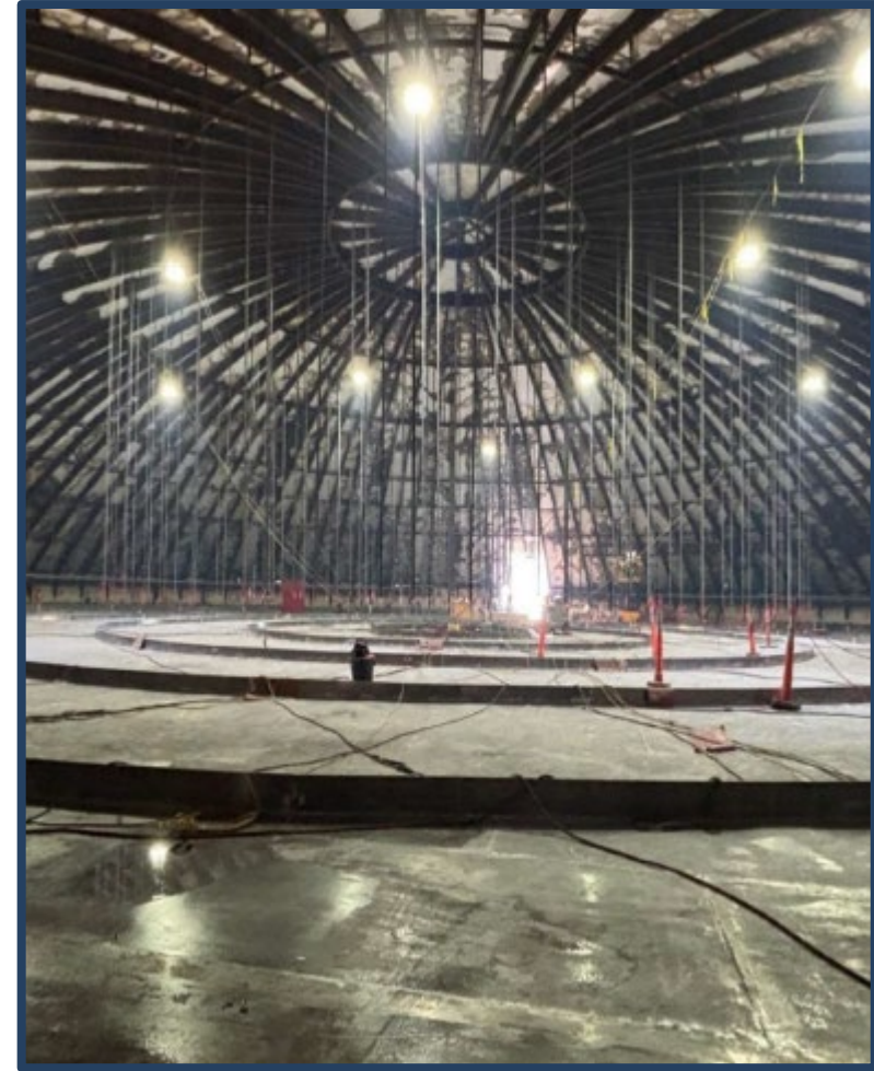
Tank 1 suspended deck construction, June 2025
