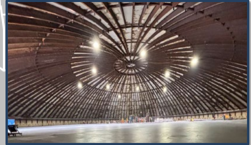
Tank 1 interior, June 2025
